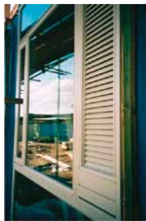
Timber framed windows and louvered ventilation
