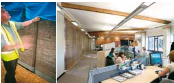
Earth-rammed spine wall during construction (left) and after construction (right)
